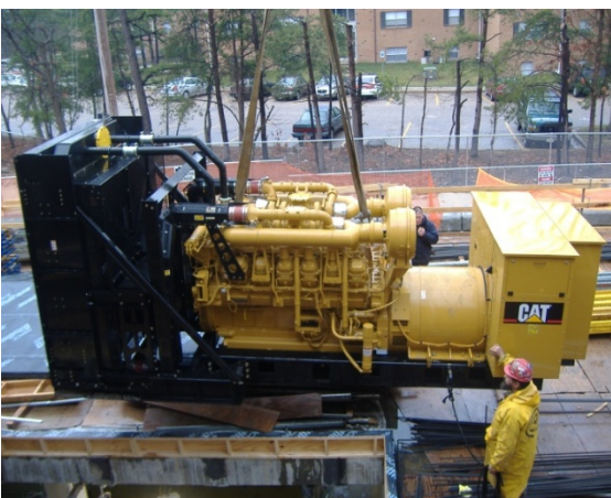
Figure 5: Image of Generator
