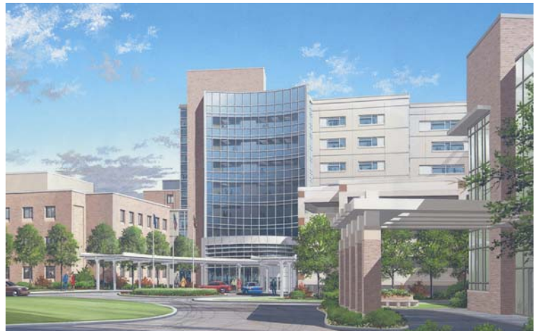
Figure 2: Image of Building Facade
