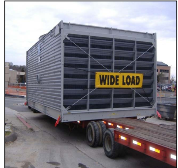
Figure 4: Image of Mechanical Cooling Tower
